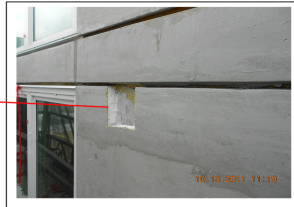
22 6 th floor EPS cut to perform test
