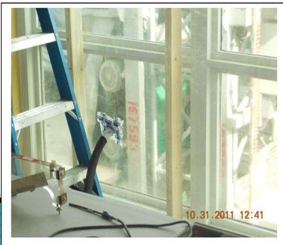
7 9 th floor window water test
