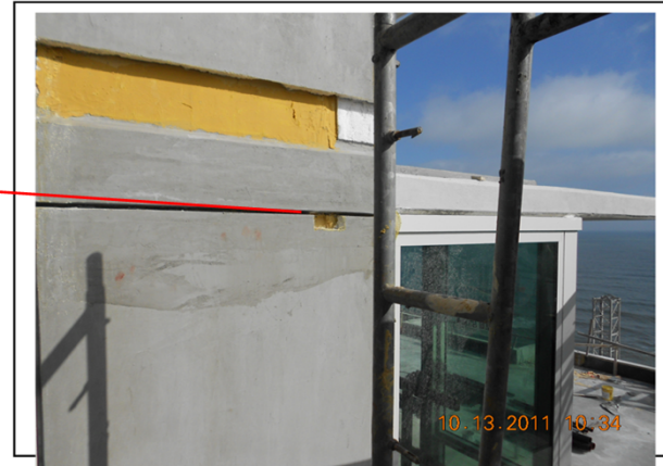
14 11 th floor EPS cut to perform test
