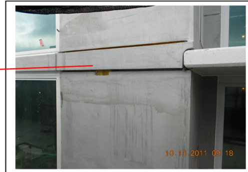
4 4 th floor water at joint below ok
