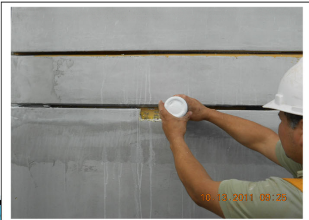
7 8 th floor water poured behind EPS
