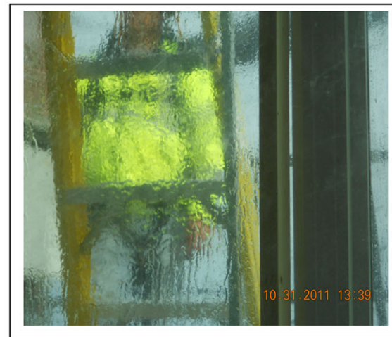
8 9 th floor window water test
