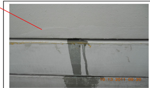
4 4 th floor water at joint below ok
