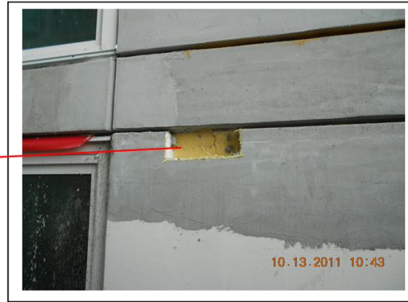
18 6 th floor EPS cut to perform test
