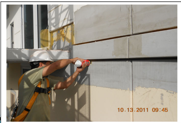
11 4 th floor water poured behind EPS
