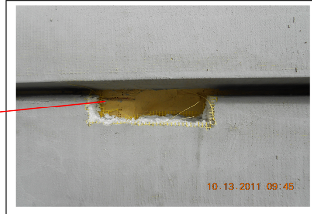
10 4 th floor EPS cut to perform test
