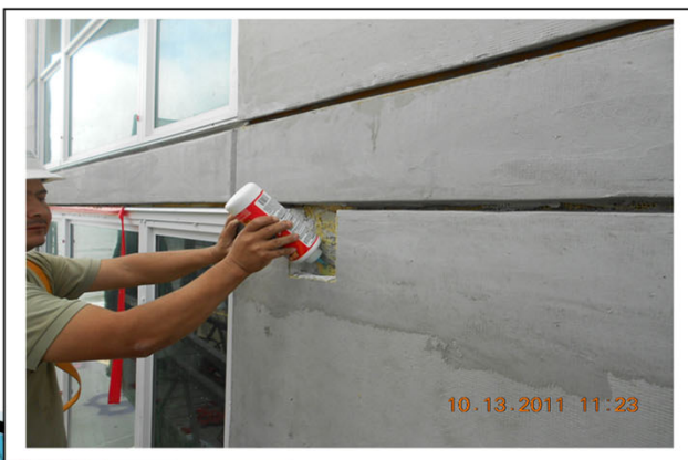
23 6 th floor water poured behind EPS
