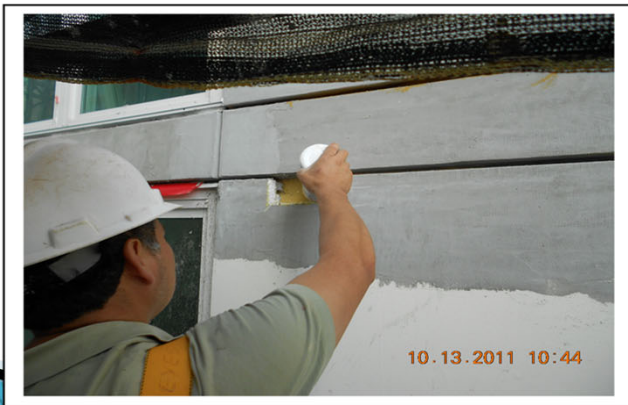
19 6 th floor water poured behind EPS
