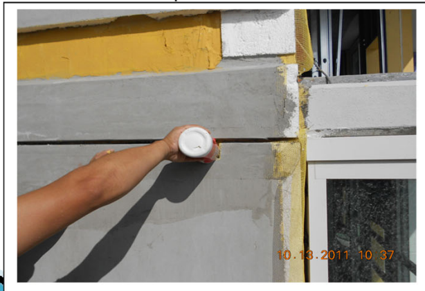
15 11 th floor water poured behind EPS
