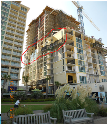
South – AREA INSPECTED
