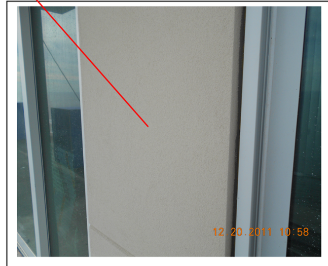
8 18 th floor finish coat ok
