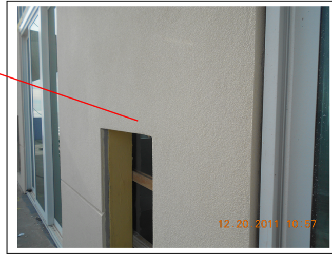
6 18 th floor finish coat ok
