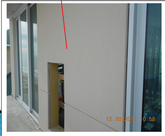
7 18 th floor finish coat ok
