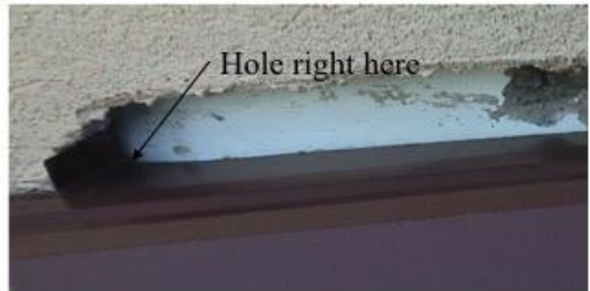
“Mock” kickout at metal roof
